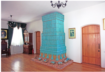
Fig.3. Reconstruction of the early 18th-century tiled heating stove at the residence of Judge General Vasyl Kochubei in Baturyn. Photo by V. Mezentsev.
